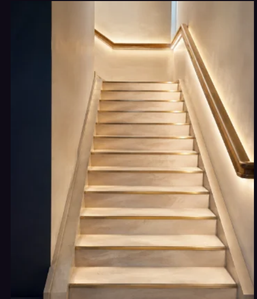
FEATURE STAIRCASE — CONCEALED HANDRAIL LIGHTING
